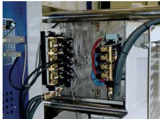
*Correction of the mold temperature by addressing the individual cooling circuits of the WITTMANN WFC: Water Flow Control.*
